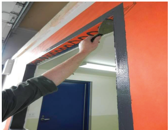
Use VAPROLIQUI-FLASH as a liquid flashing membrane in rough openings of structural walls.
