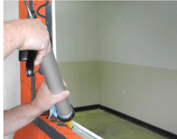
Apply using a profesional caulking gun.
