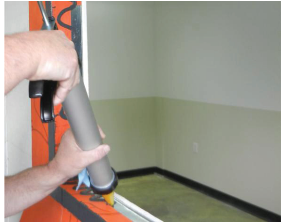
Apply using a professional caulking gun.
