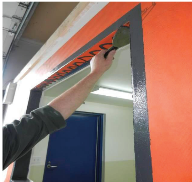
Use a DRY joint knife, trowel, or spatula to spread.
